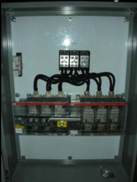
ABB Manual Transfer Switch 800 Amp Fused
